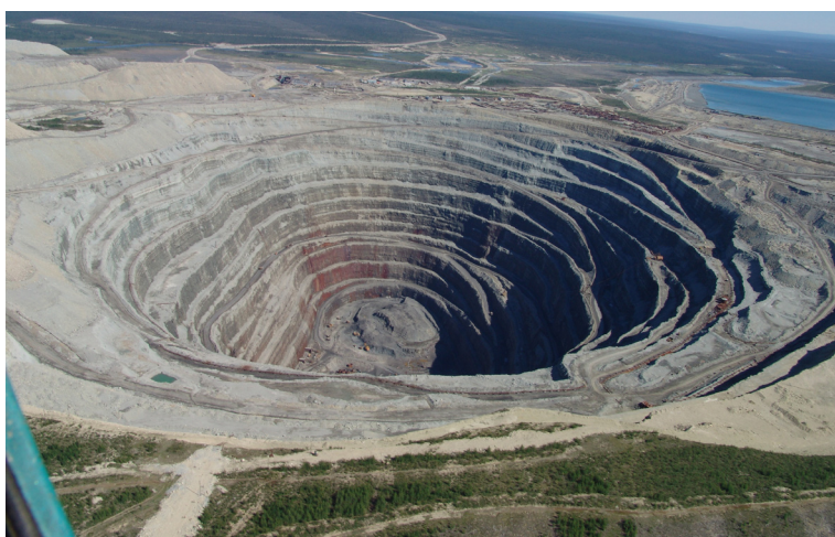
There is a definite physical limit to the depth of open pit mines
